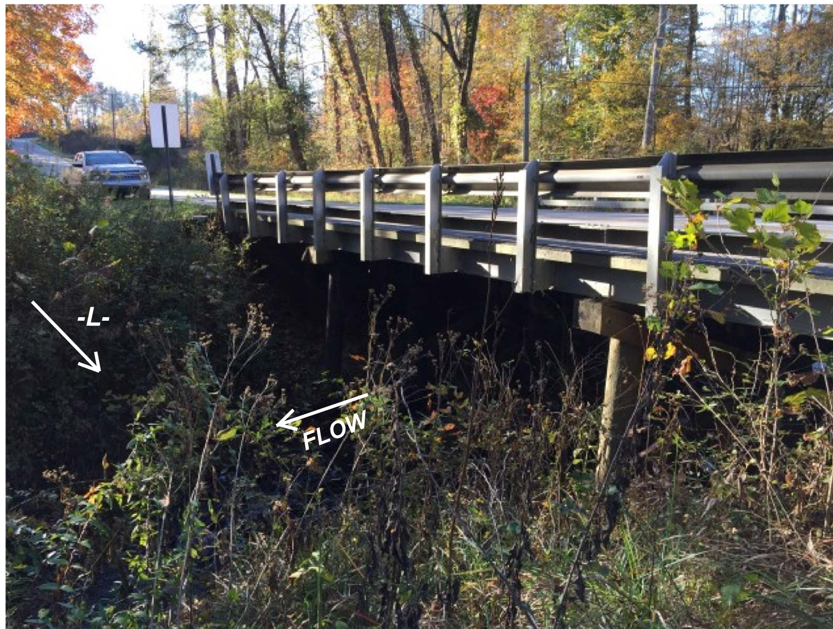
PHOTOGRAPH NO. 1.: VIEW LOOKING SOUTH
